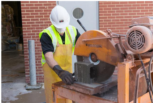
Cutting block using water to control the dust
