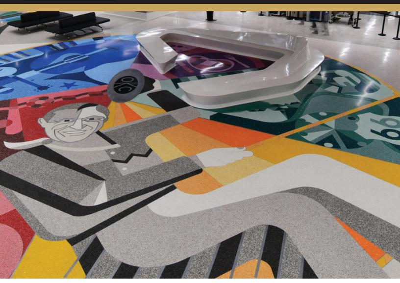
The majority of terrazzo projects installed today are the thinner-set epoxy system, and that number has grown exponentially over the past few decades. Fewer cement-based installations are specified, though the traditional sand-cushion system can be the right option for specific situations.
