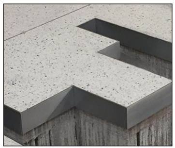
"It's not every day you work with a big rough hole in the floor with some blocks around it with crudely finished dimensions," Mr. Goldstein noted. Creating the substrate involved meticulous work in making it dimensionally correct, square and plumb.
