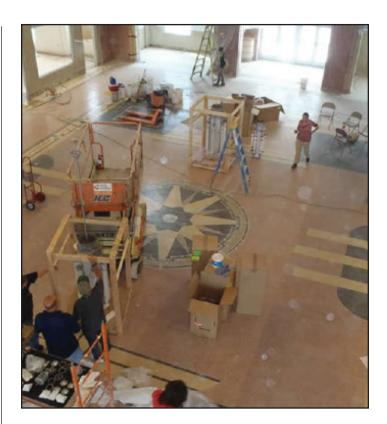
Terrazzo floors around the city were found intact. Many were in older buildings, including the train station terminal. If structural collapse or large equipment falling had chipped or gouged them, these floors were reparable. As in the airport, most required nothing more than polishing and refinishing.
